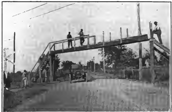
One of the numerous small bridges adding to safety of the course
